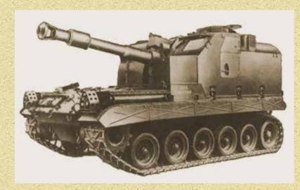
The initial design of the T99E1 had an enclosed gun compartment on special request of the US Army in order to protect the crew for battlefield dangers.
